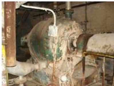
42 Inch Sprout Refiner Front
