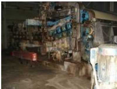
Twin Wire Press Front Side
